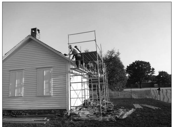
Visitors to Hoggatt School will be able to view the new wood shake shingle roof installed last summer (above), funded in part with a State of Iowa Country Schools Grant, funded by REAP, Resource Enhancement And Protection. The repairs were made in keeping with the historical character of the structure.
